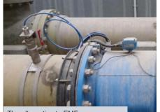
The alternative to EMFs. Installation without removing the EMF
