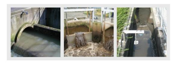
The hydraulic methods are used to calculate flow **Q** from level **h** considering a **Q - h relation**.
