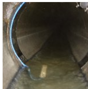
Hydrostatic measurement – for installation on the side of channels tending to sedimentation e.g. submergence detection
