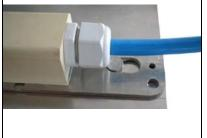
... until it is locked (flush to plate)
