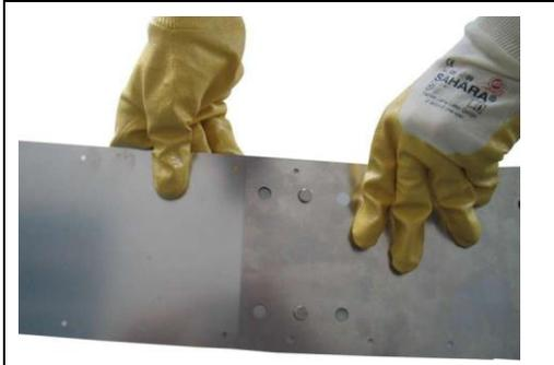
Insert the spigots of the base plate into the holes of the extension sheet.
