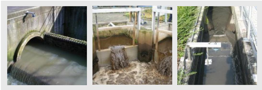
The hydraulic methods are used to calculate flow  $Q$  from level  $h$  considering a  $Q - h$  relation.
