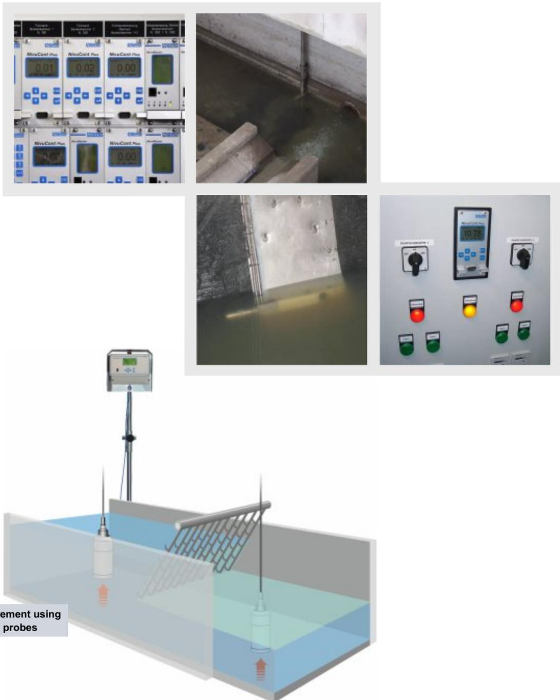
Comparative measurement using hydrostatic pressure probes
